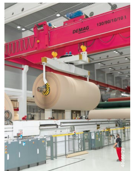
Demag process crane with motor-driven rotating reel spreader
